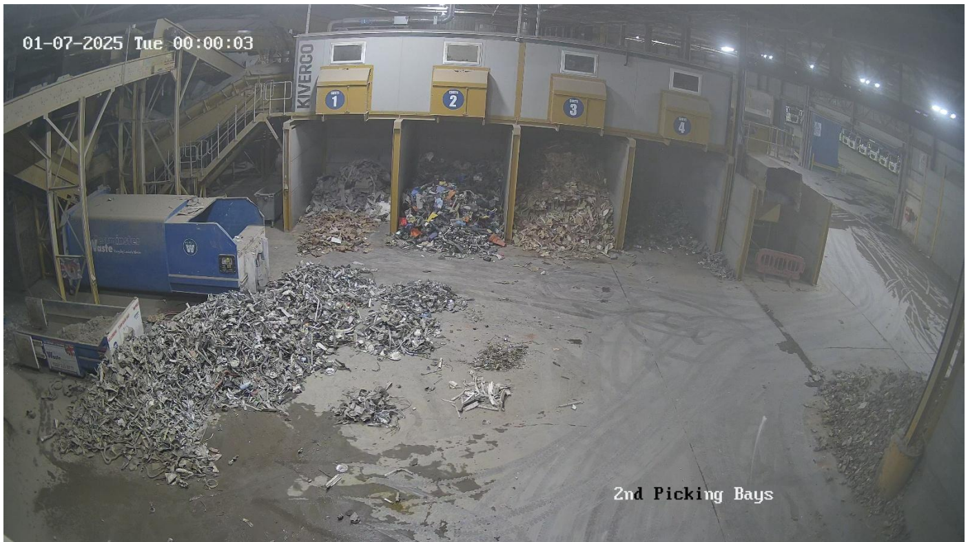
Various storage areas of segregated waste streams under picking line.
