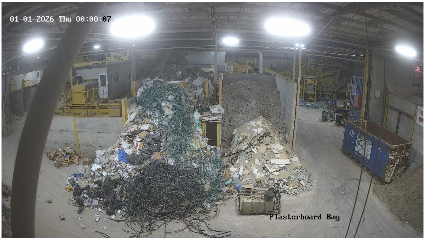
Various storage areas of segregated waste streams.
