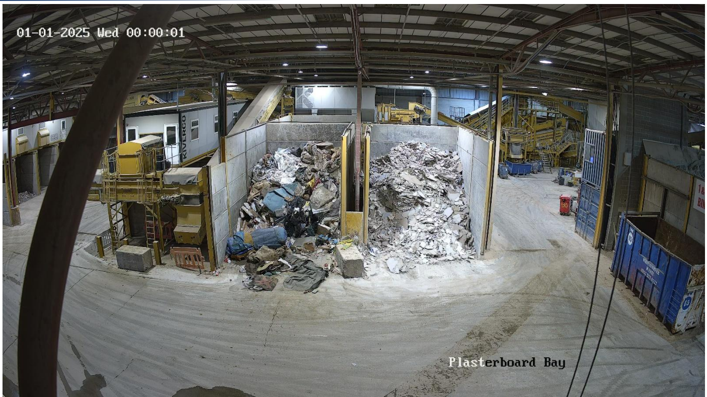
Various storage areas of segregated waste streams.
