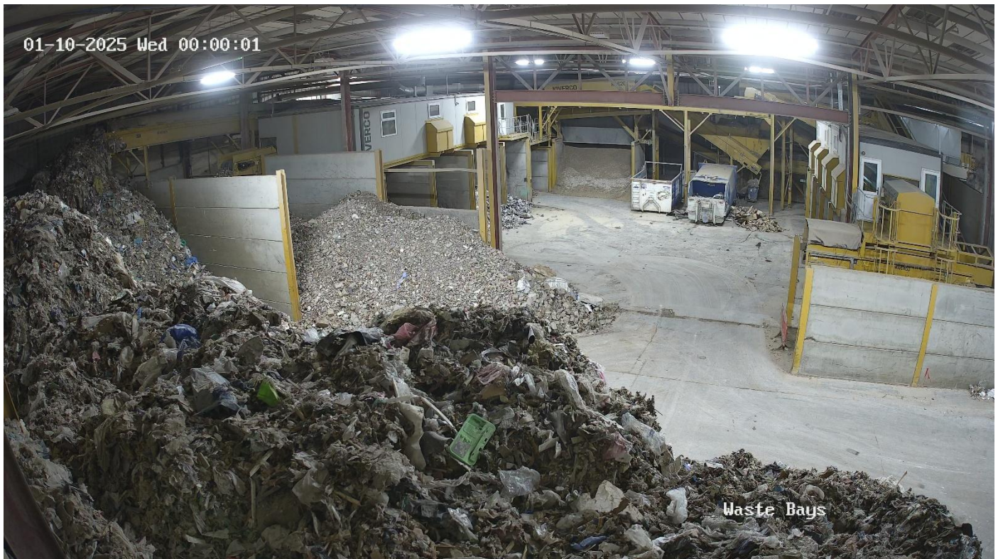
Various storage areas of segregated waste streams.
