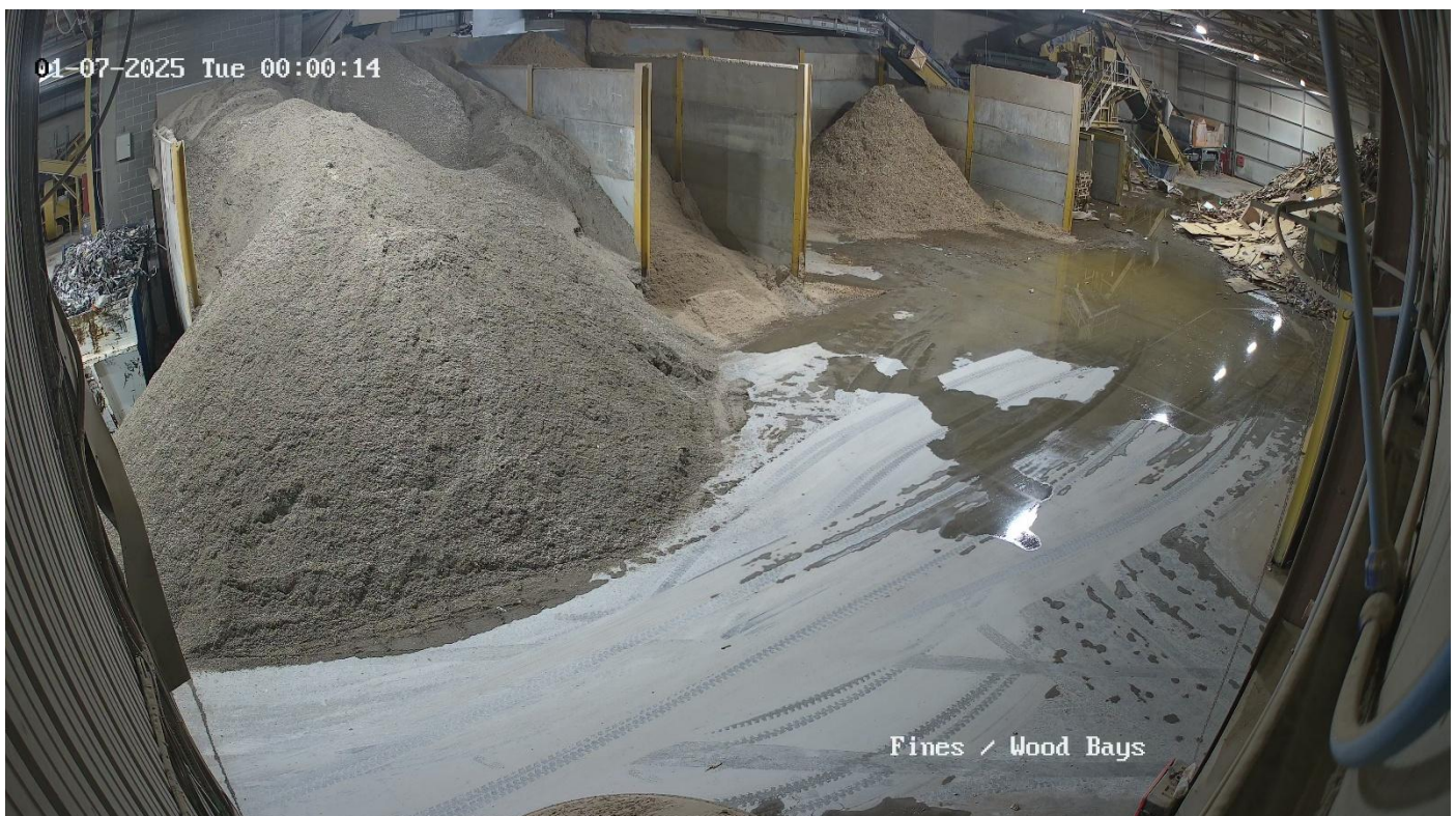
Various storage areas of segregated waste streams.
